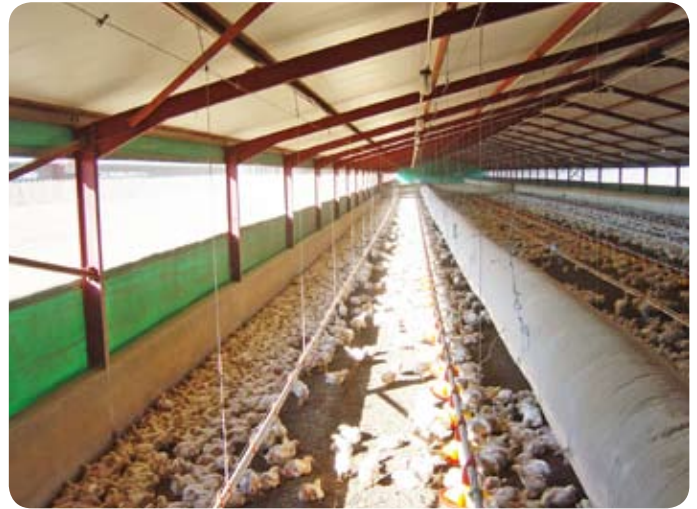
Naturally ventilated house.
